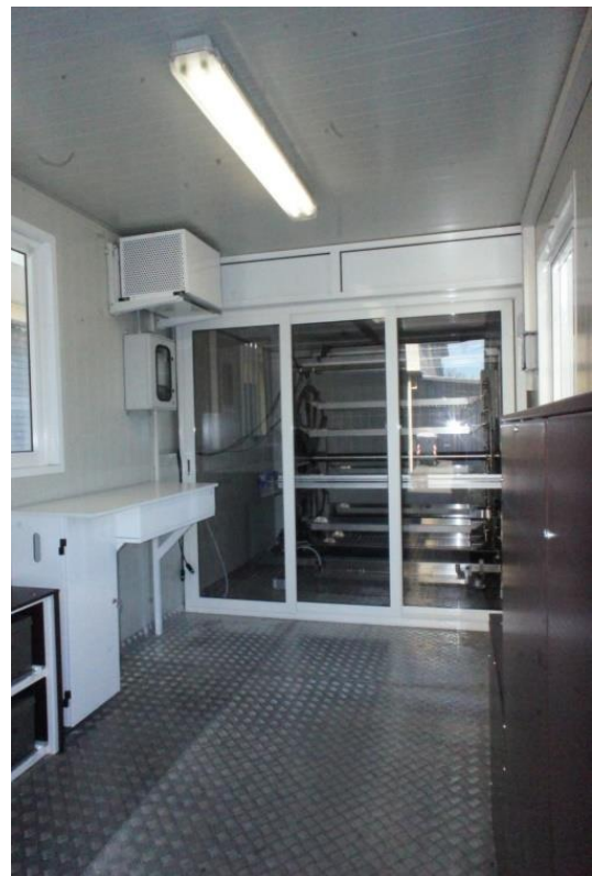
Figure XI –Architecture of Zephyr system, the growth unit inside the container and a screenshot of the control software
