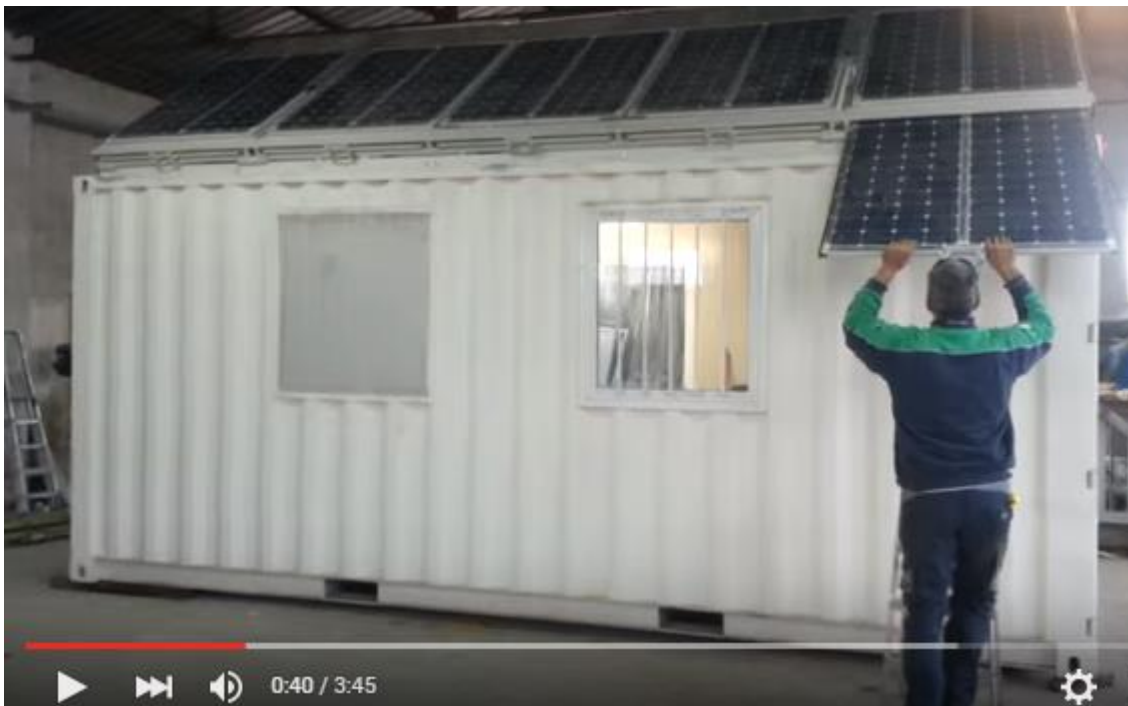
Figure 2: PV panels installation
